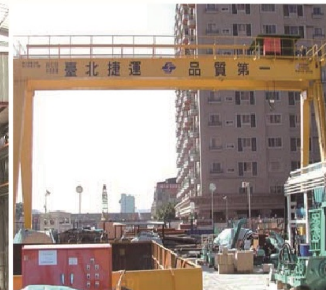
2005 Taipei MRT 10 tons crane
