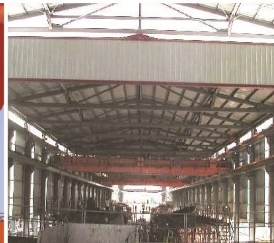
2001 Taiwan High Speed Rail mobile plant
