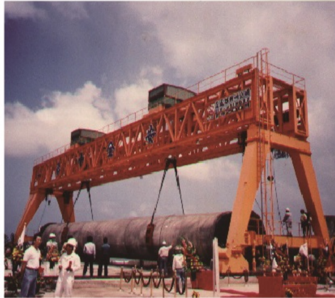
1988 Bali, Taipei 200 tons crane project
