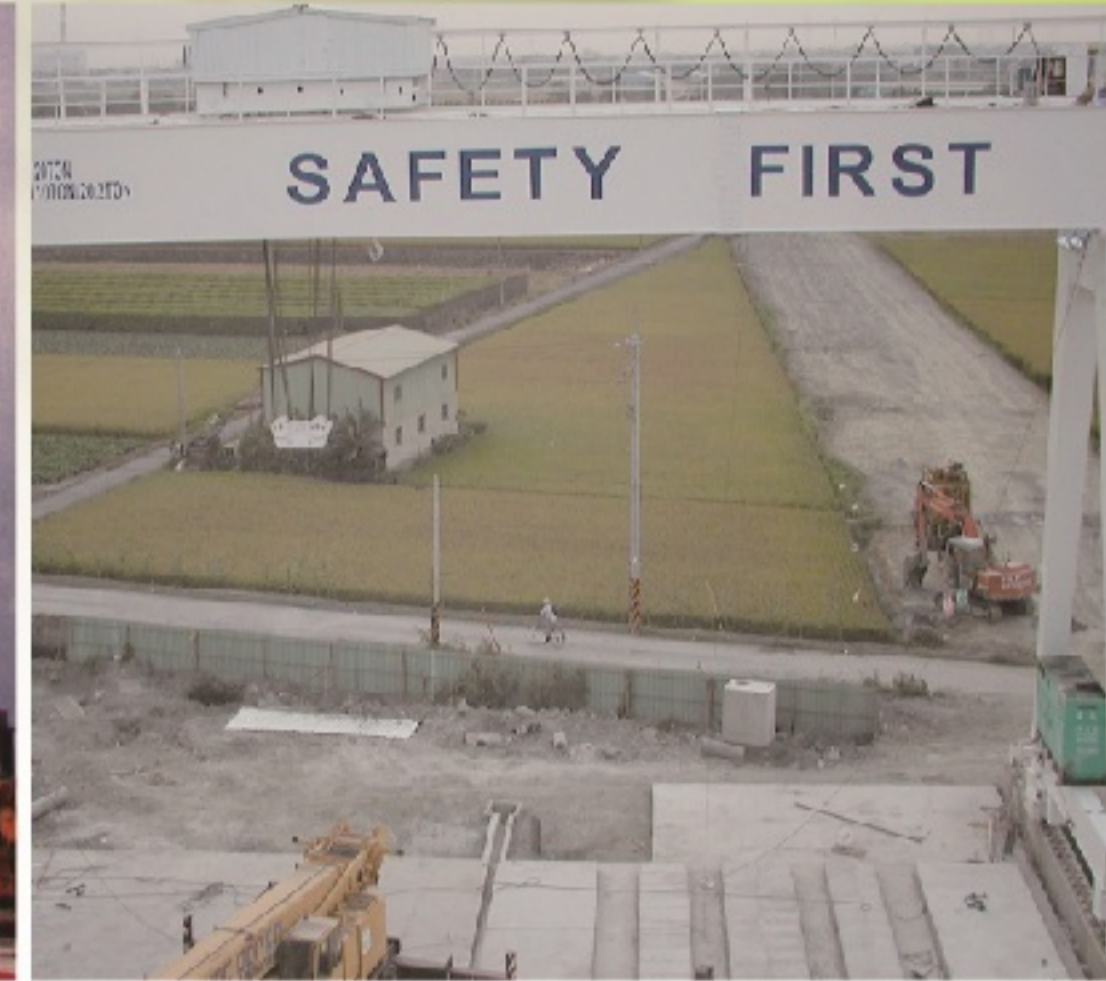
2001 Taiwan High Speed Rail 100 tons gantry crane
